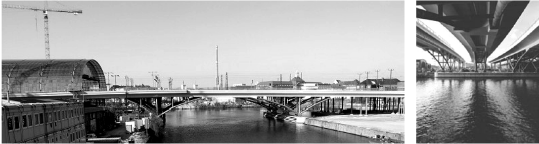
Figures 1 & 2: Humboldthaven Railroad Bridges at Lehrter Bahnhof - Berlin, Germany
